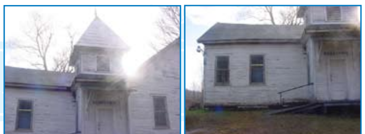
Beartown School before paint and repair work
